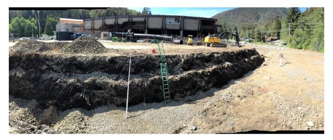
it towards the final tie-in point where last May, the 42-inch wye joined with the 36-inch ductile iron raw water main adjacent to the Ketchikan Charter School. The joint as assembled with the 36-inch main to the left is shown in the photograph below.
